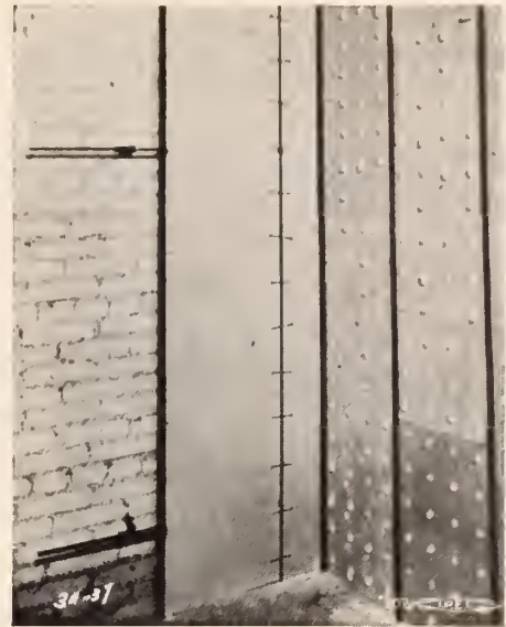
Photo No. 3. Angle of Room showing Insulated Outside Wall (see detail No. 7) and back view of perforated Rocklath Partition (see details 1, 2 and 3 and photo No. 1.)
